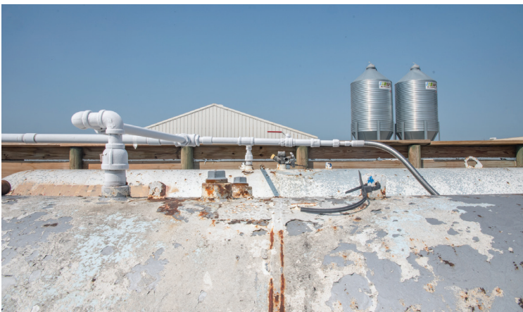
LP tank piping frosted over
