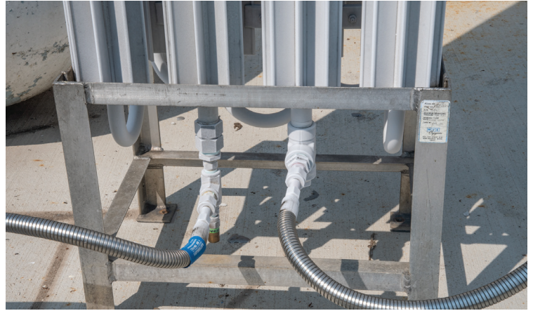
Frosted input and output connections on vaporizer
