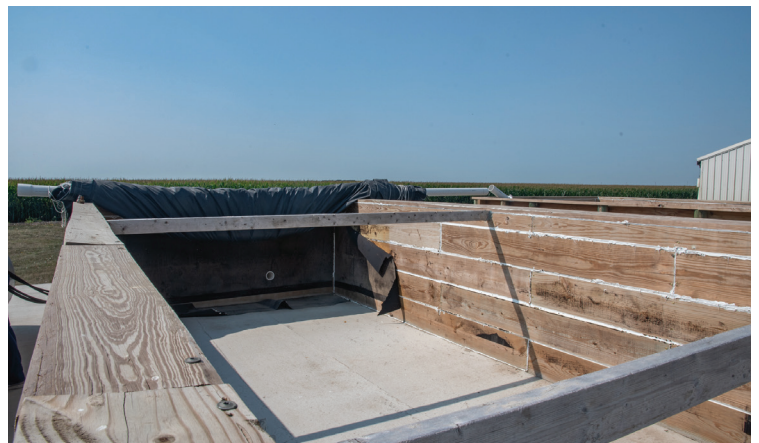
Wooden boards to hold tarp
