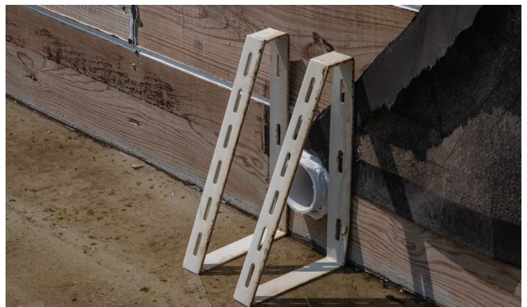
Pipe protective cover to prevent pigs from blocking CO 2
