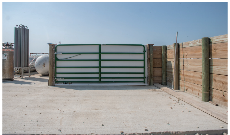
View of closed gate to chamber 1
