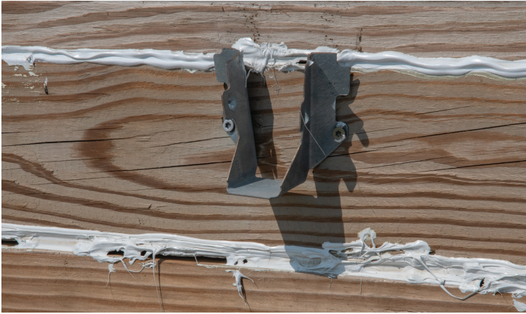
Attachment to hold wooden boards to support the tarp
