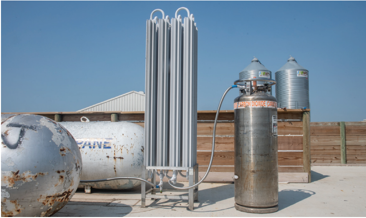
View of vaporizer and single CO 2 tank
